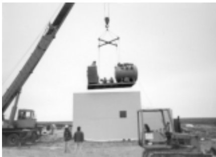
The vacuum station for Beach Road MUD's vacuum system is the same as pictured above. The photos at left show construction of the vacuum station building, the station arriving at the community on skids, and the station being lowered into the building.
