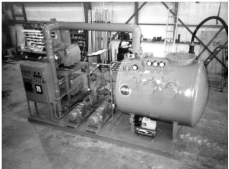
Photos Courtesy of Airvac, Inc.
