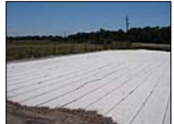
A drip irrigation system is a type of micro irrigation system. The system is operated to maximize the amount of unsaturated flow. This is accomplished by frequent, low-pressure applications of the treated wastewater within the biologically active zone. Under unsaturated flow conditions, there is improved renovation, and aeration of the wastewater.
