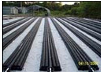
Multi-Pipe units allow for exceptional soil contact and are engineered with holes and slots, allowing it to collect and disperse the effluent as it passes over the corrugations in the pipe.
