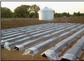
The Low Pressure Dosing (LPD) System works well in soils in which gravity flow, conventional systems have failed. Such soils are typically tight clay soils in which there is no evidence of a seasonal high-water table (as evidenced by mottling or discoloration of the soil).
