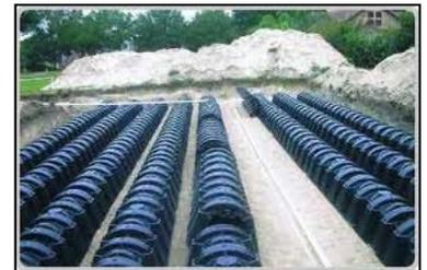
The chambers treat more effluent, more efficiently, in a smaller area. They also have a much greater storage volume and offer a very large surface area for effluent infiltration into the soil and can be installed in tight, sloped and curved areas creating less site disruption to landscaping.
