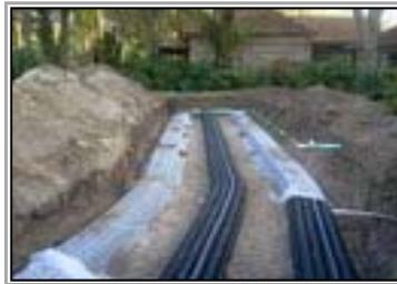
The terms Gravity or "Conventional" Septic systems refers to the simplest type of septic system where the water flows (by gravity) from the house to the septic tank and then to a Distribution box or manifold and finally to a trench or bed type absorption field (drain field) where it soaks into the ground.
